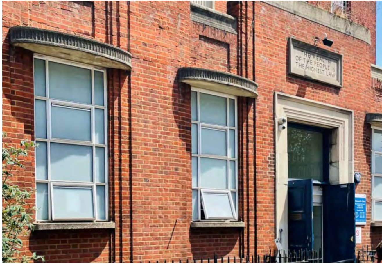
A Walworth Road Clinic- a finely proportioned brick facade
